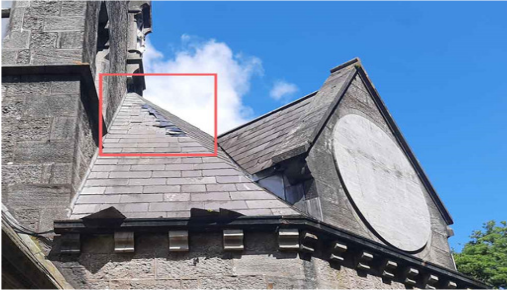
Area of slate loss at chapel apse roof
