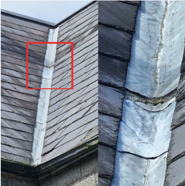
General view and close-up view of slipped valley gutter
