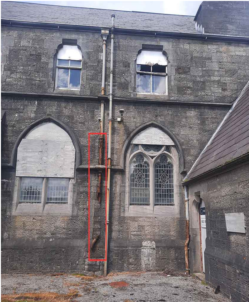
Replacement downpipe at RWP 2 - new bend and shoe required - South elevation
