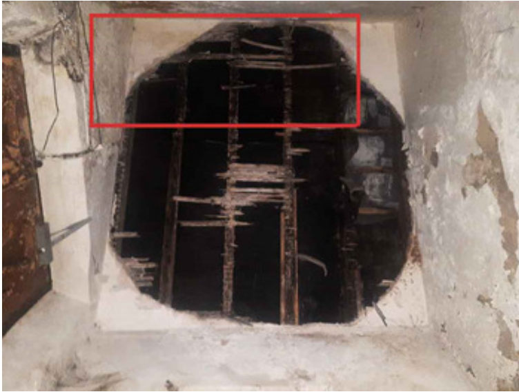
Underside (ceiling) of Chapel Porch Roof – showing rafter ends to be repaired
