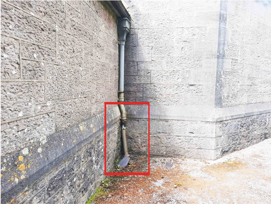
Replacement downpipe at RWP 4 - Sacristy - new shoe also required - South elevation
