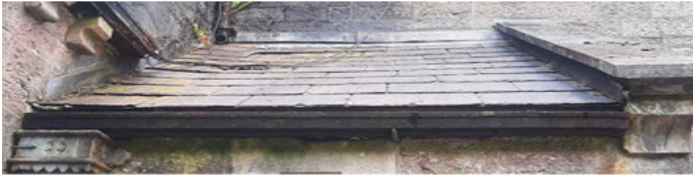
Close-up of damage at Chapel Porch Roof - section of surviving historic gutter also shown
