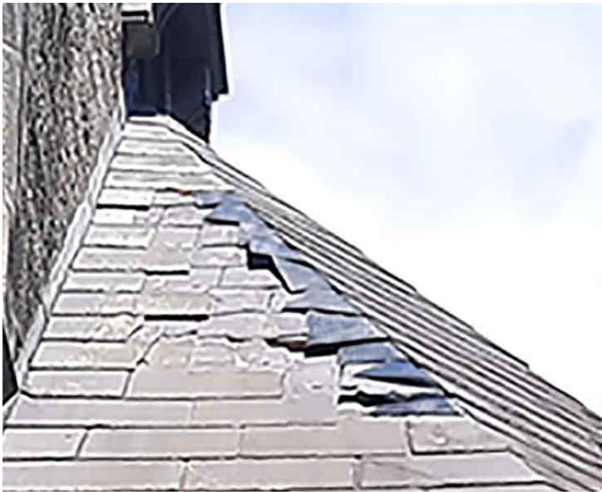
Close-up of slate loss at chapel apse roof
