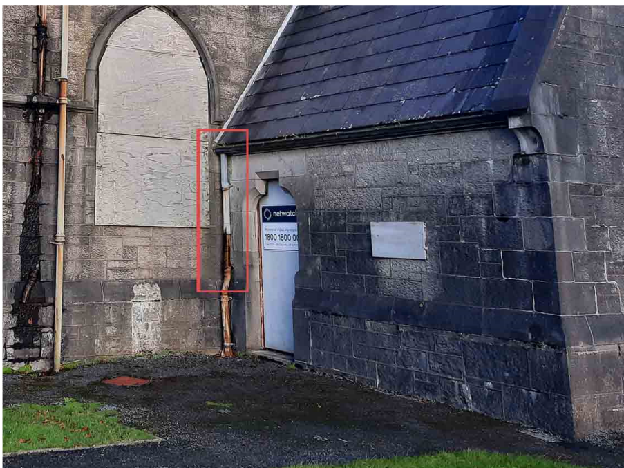
Replacement downpipe at RWP 3 - Sacristy - South elevation
